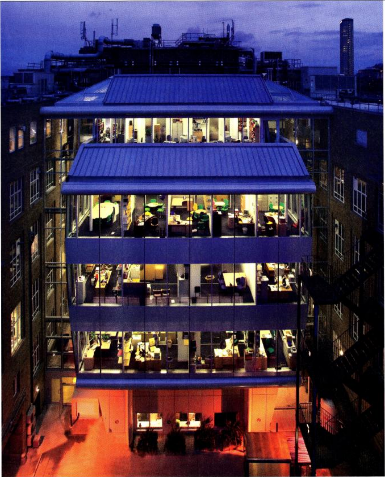
2. Photovoltaic panels are only the most visible elements of the sustainability strategy
